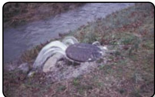
Stormwater infiltration causes sanitary sewer to overflow.
