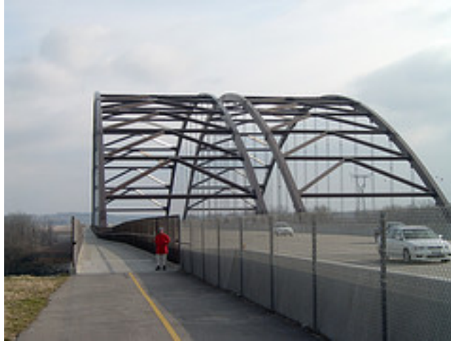
Page Avenue, Missouri River Bridge bicycle/pedestrian path, St. Charles, Missouri
